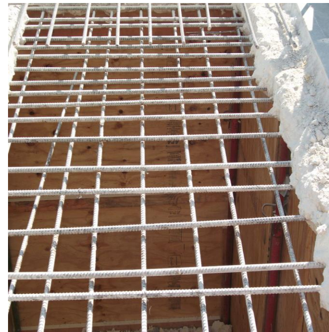
Missing Rebar
