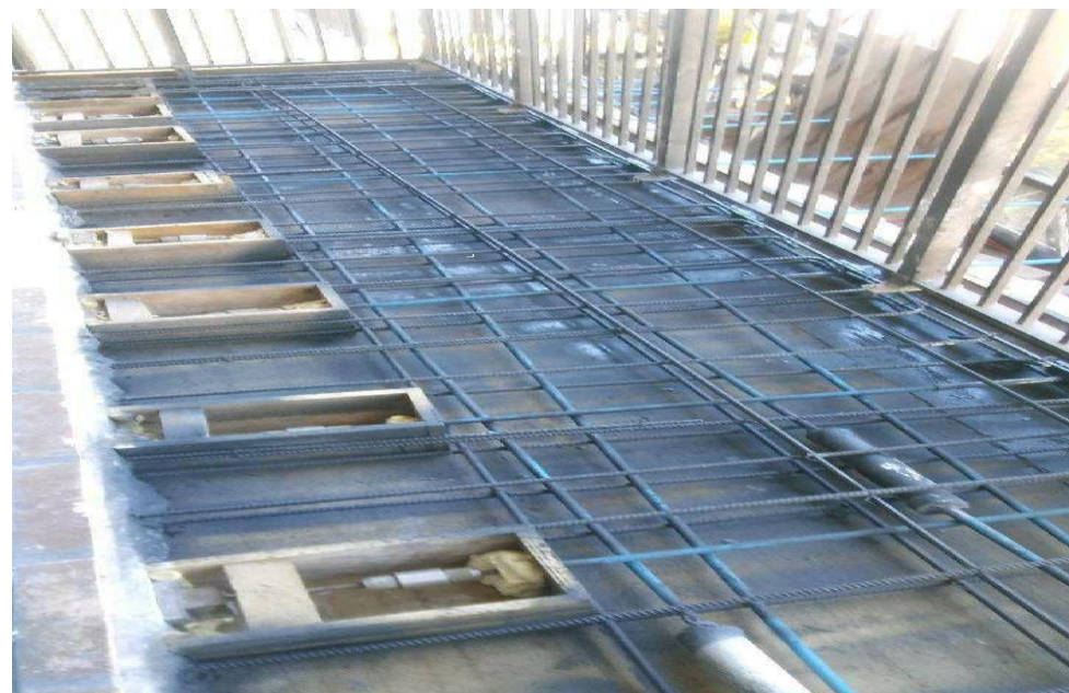
NEW Post Tension Cables, Anchors, & Reinforcements.
