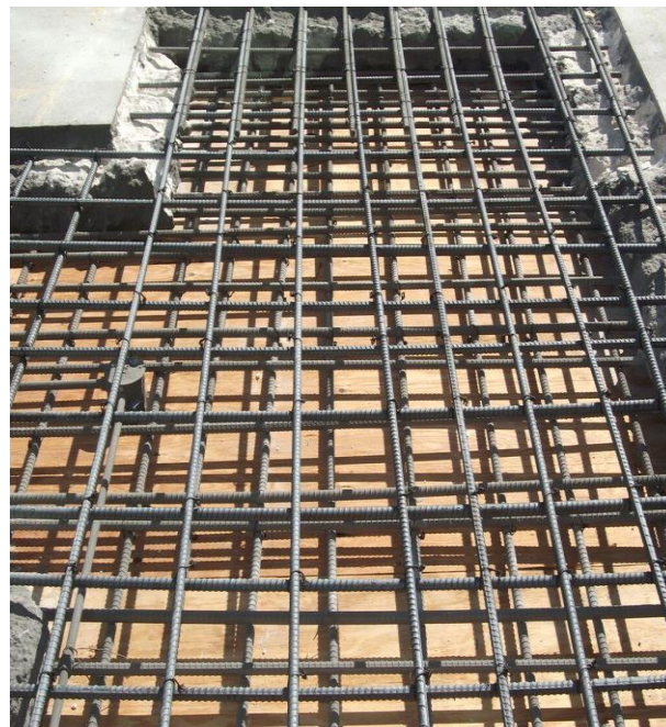
Added Rebar and clean
