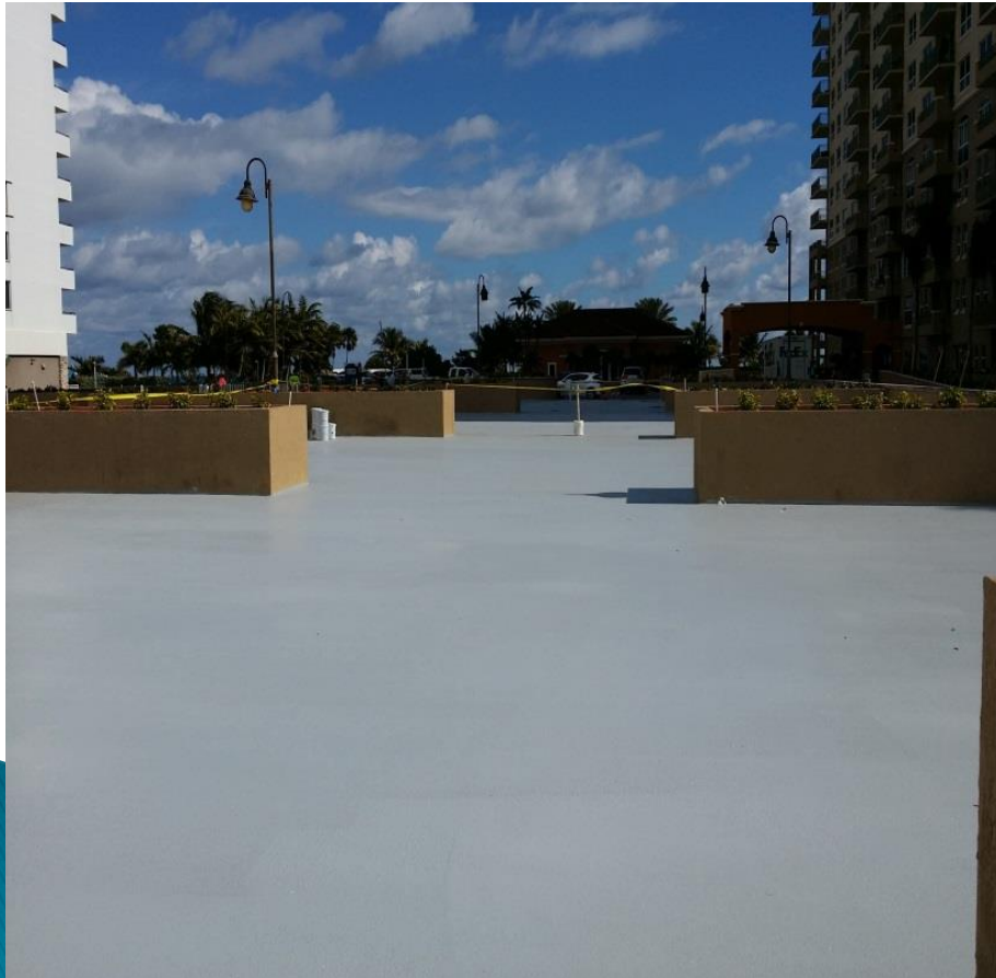
New Waterproofing Applied
