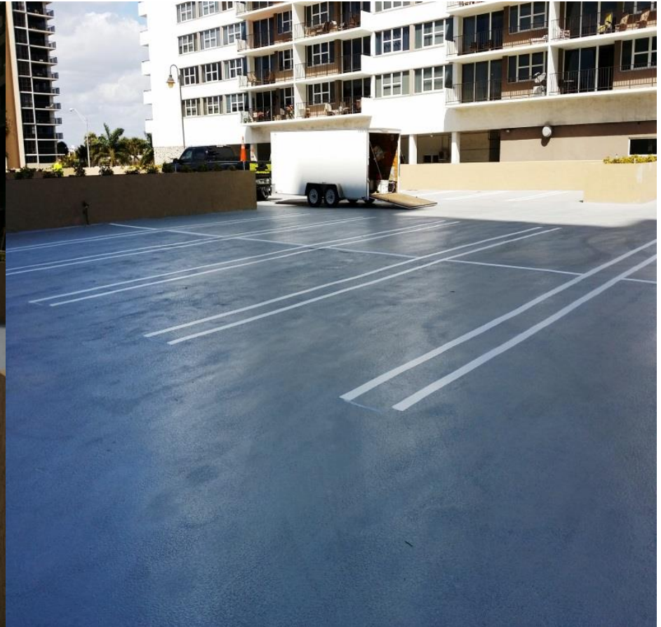
Project Complete with Parking Stripes
